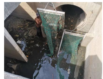
Securing pins to release/retain the rubbish
