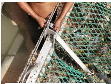
Take off the securing pins for maintenance
